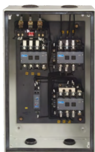
Interior View of MU FASD
